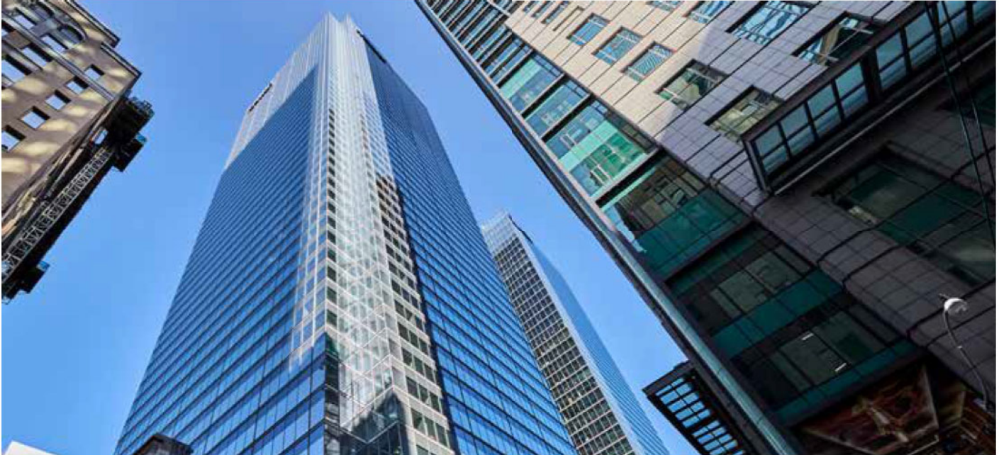
Look up! The Bay Adelaide Centre was fabricator Walters Inc.'s first foray into high-rise construction.
