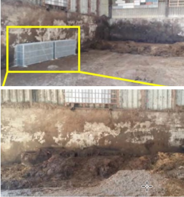
Test conducted in a cow farm - manure storage area
